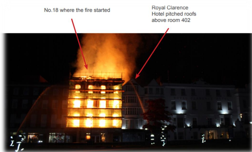
Figure 5 - Fire at No.18
